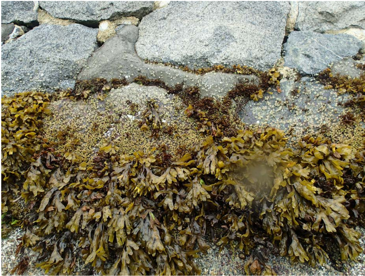
Upper Intertidal - seawall
